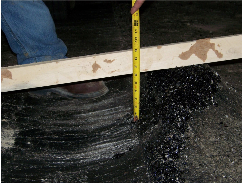
Figure 4-12 QW lane failure first experiment
