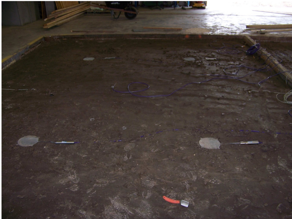
Figure 4-4 Pressure cells installed in subgrade
