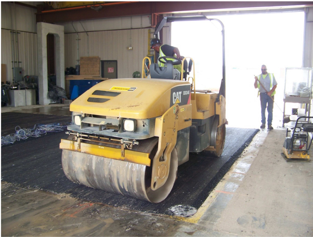
Figure 4-9 Asphalt compactor
