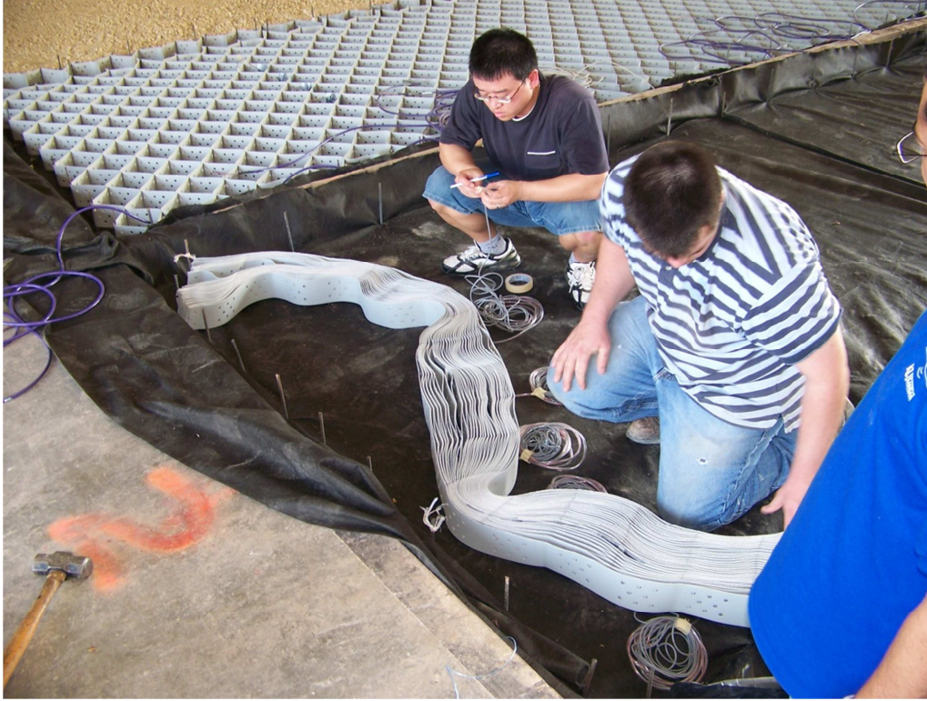
Figure 4-5 Geocell installation
