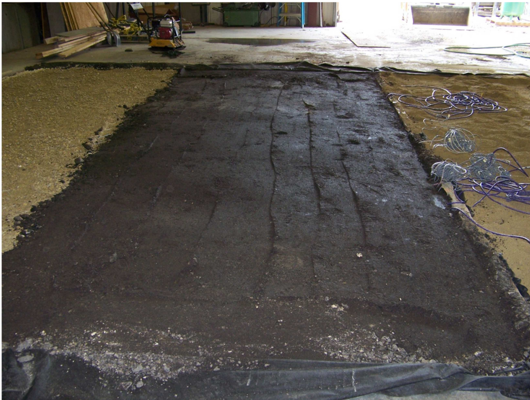
Figure 4-6 Infill after vibratory plate compaction
