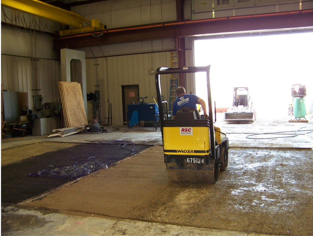
Figure 4-7 Roller compaction of infill
