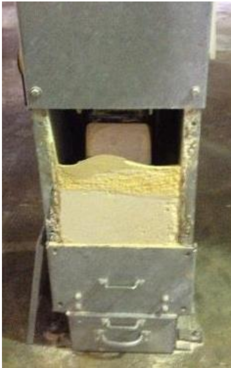
Figure 1.6 Bucket elevator with potential contamination
