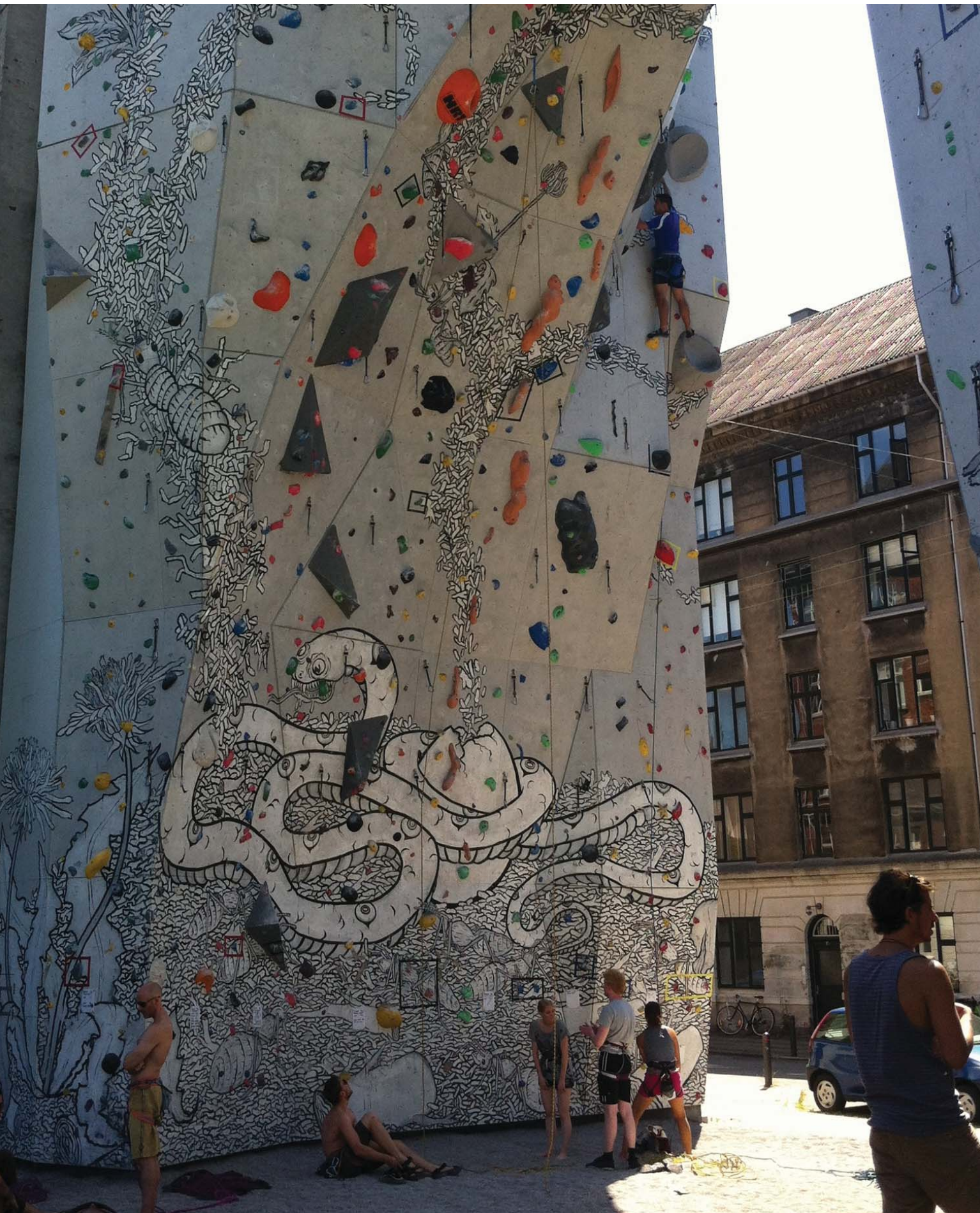
climbing wall in Copenhagen, Denmark (author 2014)
