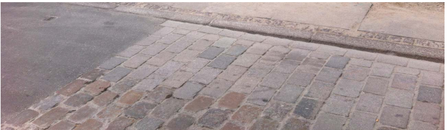
Fig. 52. Smooth pavement implemented on bumpy cobble stone streets in Copenhagen (author 2014)
