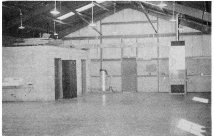
The north end of the enclosed building showing the water pump, heating system, and rest rooms. This building is used for meetings as well as for the 4-H Fair.
