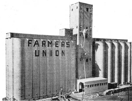
FUJA Terminal Elevator Topeka, Kansas
