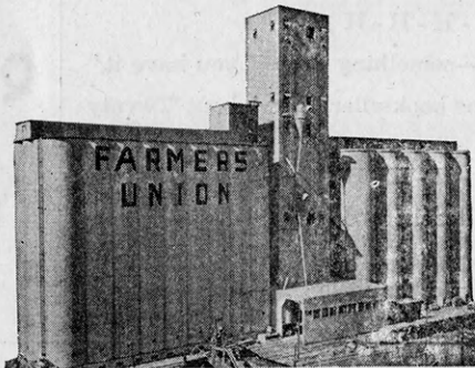
FUJA Terminal Elevator Topeka, Kansas
