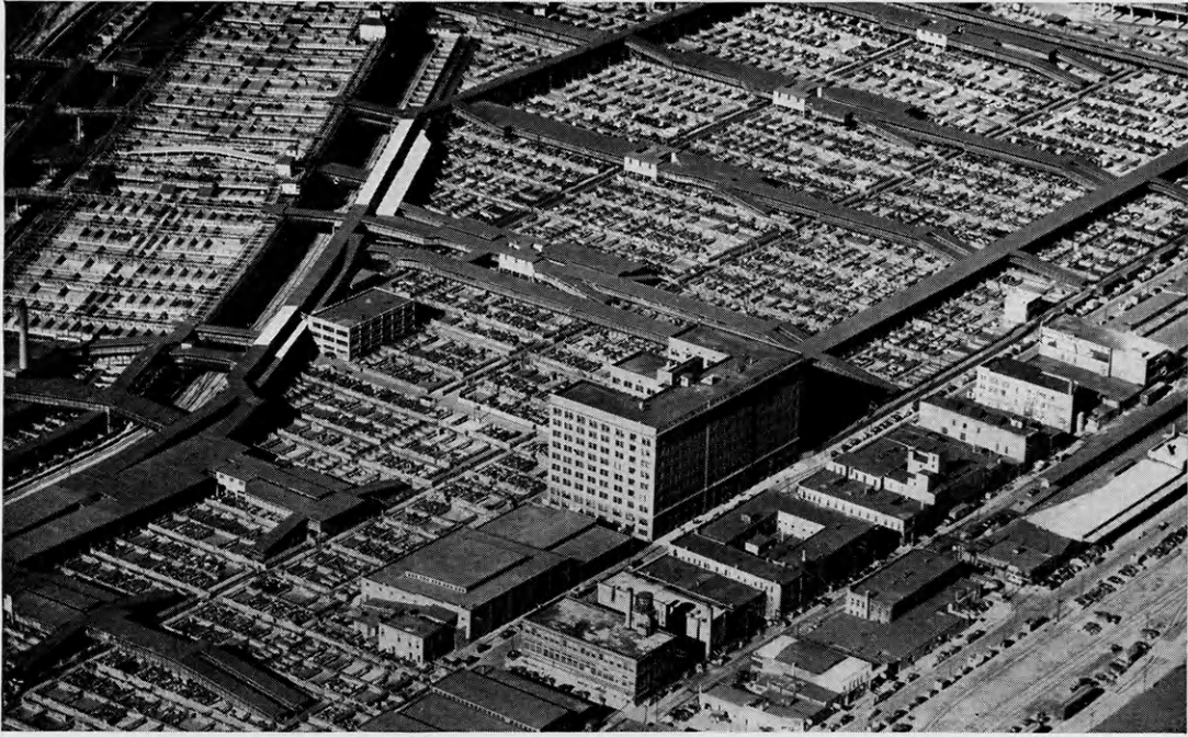
● A Recent Aerial View of the Kansas City Stock Yards
