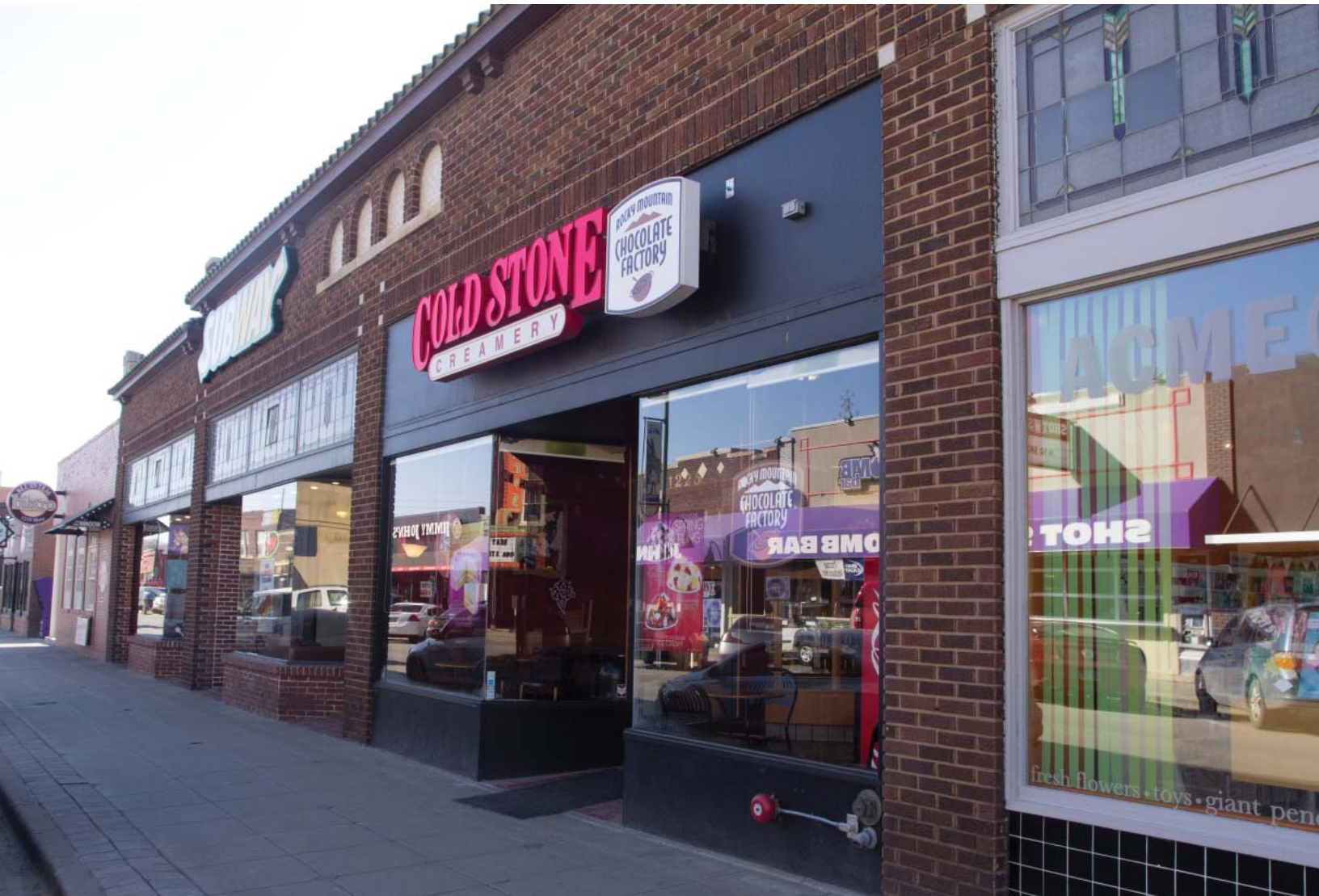
Figure 2-15 High Quality Building Facade of Moro Street
