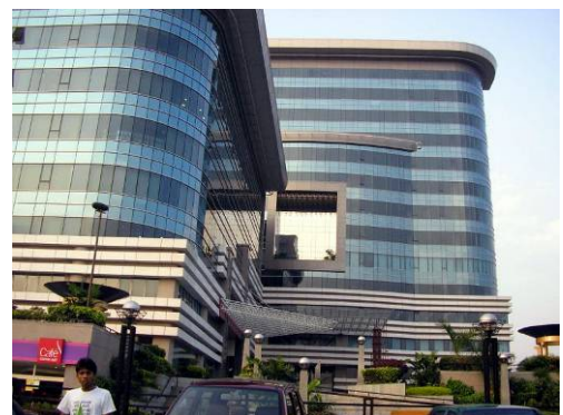
Figure 71: Corporate building, Sector 5, Salt Lake
