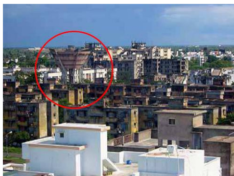
Figure 70: Water tanks act as landmarks in Salt Lake City blocks
