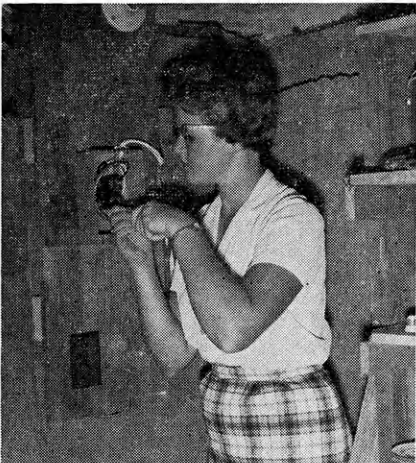
Linda puts the fuse box in the basement of the bunk house which she wired.
