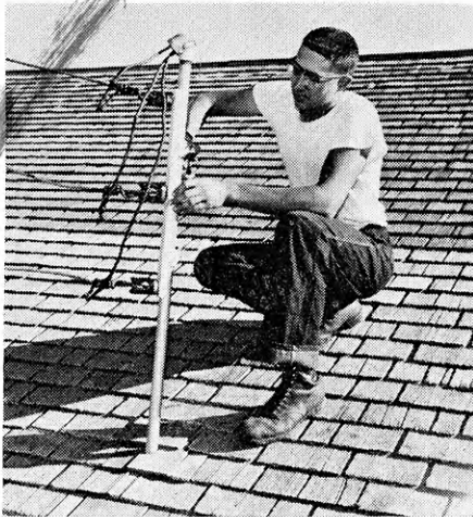
Making his own roof jack from a pipe, Bernard ran electric service to the farm work shop.
