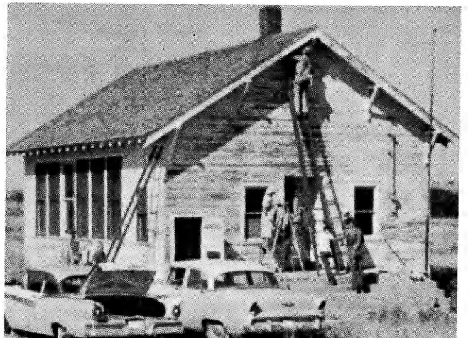
Plum Creek members and parents, Cheyenne county, gave the Hackberry school, now used as a community center, a thorough going over recently. Renovation included paint, new windows and doors, mowing, scrubbing and waxing.
