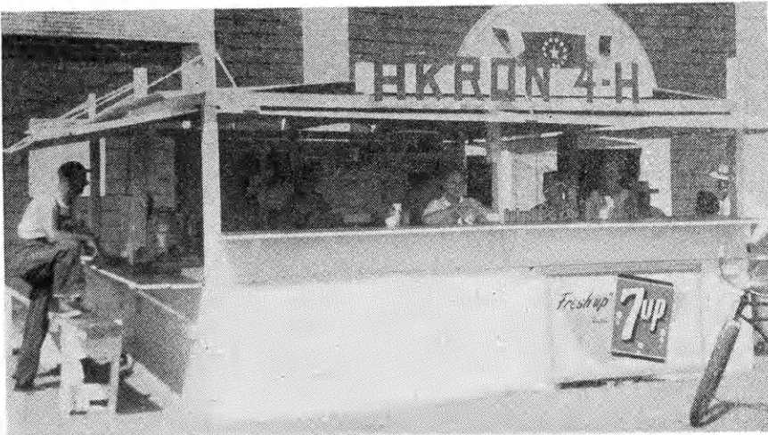
A new paint job and some needed additions were added to the Akron 4-H Club's food stand before the Cowley County Fair. The Junior Leaders worked on reroofing the stand and putting a floor in it. They also built two six foot extensions onto it.
