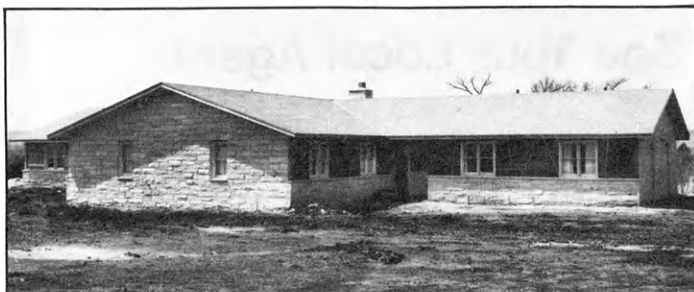
Construction of Finnup Cottage at Rock Springs Ranch completes the year-round sleeping accommodations at the facility.
