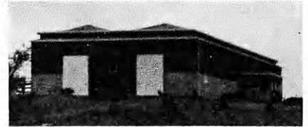
Showing a back view of the new Christy stables at Rock Springs Ranch, the building is made of concrete and redwood. The fireproof concrete roof is the only one of its kind on a farm building in the U. S. The picture at right shows a front view.
