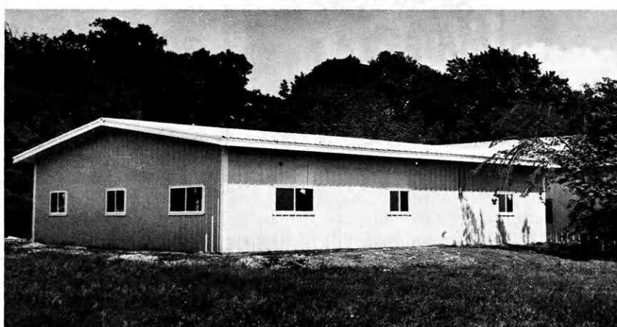
The newest building at Rock Springs Ranch is the Frye Workshop building. The 40 by 60 foot structure will be used as a maintenance and repair shop.
