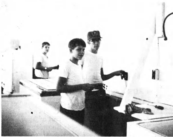
Wiring a receptacle on one of the new circuits installed in the 4-H exhibit building are Mark and Eddie Crum-packer and Ralph Ulery. Eight new circuits and nine receptacles with grounds were added to accommodate the freezers used for the sale of homemade ice cream by the Crawford County 4-H Council during the county fair.
