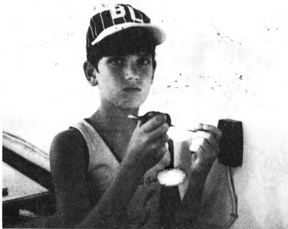
Doug Chadd is shown using a test light to check out one of the new receptacles.
