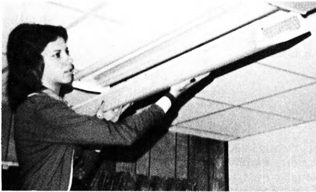
June helped put in the electricity in a new room on their house. Here she is putting up a fluorescent light fixture.
