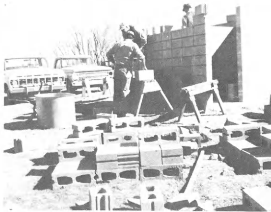
When Wright Wonder Workers 4-H Club in Ford County received a grant from Southwestern Bell Telephone Company through Kansas 4-H Foundation for building restrooms at the ball park, other community organizations were ready to help. The Knights of Columbus did construction work, shown above, and St. Andrews Parish gave $100. The 4-H members painted the building. Audrey Grasser was project chairman and Neil Salmans is community leader.
