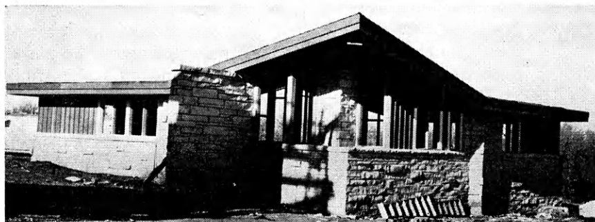
This health center is one of three buildings now under construction at Rock Springs Ranch. The nearly completed structures were made possible by a contribution from the A. D. Jellison family of Junction City to the Rock Springs Ranch development.
