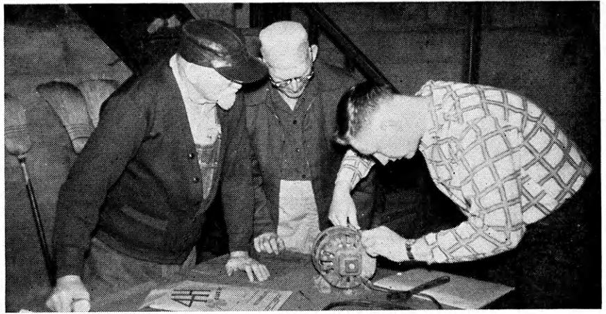
Mr. Sites and Mr. Vanetta supervise as Carl Lee Nichols starts to disassemble and clean an electric motor.
