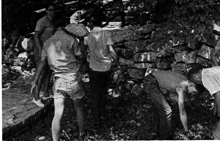
They rebuild a wall—
