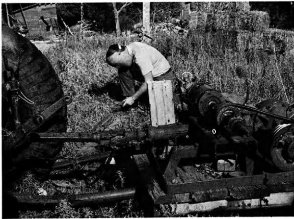
HOMEMADE WELDER —Here Albert does some welding using the tractor-powered electric welder he made in the 4-H electric project. Albert plans to join the U.S. Air Force and continue his training in electronics. Electric has been his favorite 4-H project.
