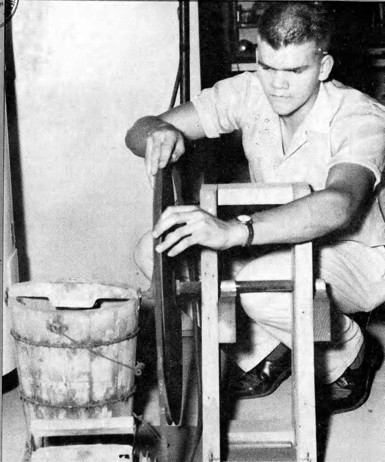
Alan Moore, Kansas 1957 Electric winner from Sedgwick county, shows the mechanism he made to hook an electric motor to his ice cream freezer. For more details on the new electric project for Kansas, see pages 8 and 9.
