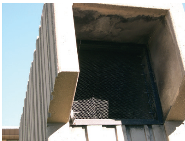
Figure 4.15: Air shafts are essential to the parking garage, but the colossal structures are daunting, September 30, 2005.
