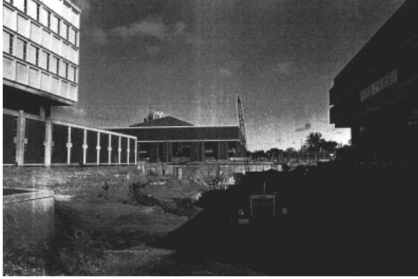
Figure 4.3: The Mall under construction to receive a two story parking garage 1972. Photo by John W. Alley with permission from the University Archives.
