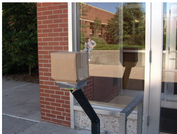
Figure 4.16: Public protection during construction at a building entry, September 30, 2005.
