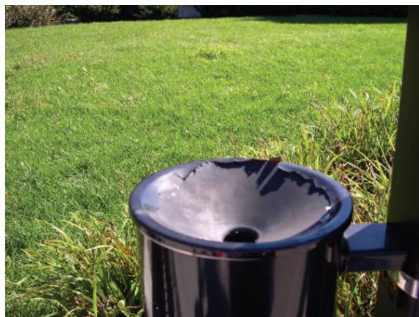
Figure 4.14: Cigarette receptacles and light posts require regular painting, September 30, 2005.
