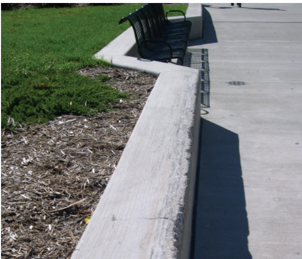
Figure 4.13: Seatwalls show wear and tear due to skateboard use, September 30, 2005.
