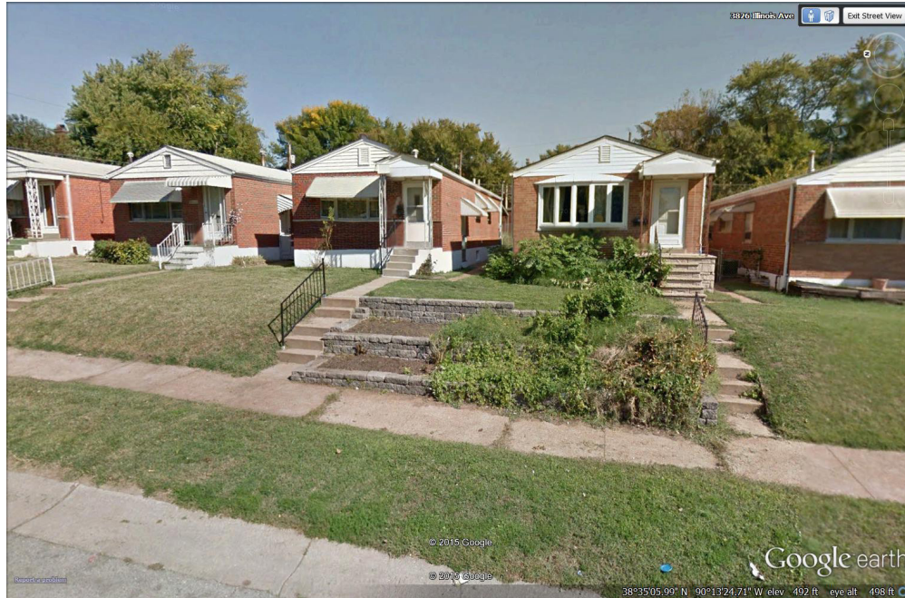
Figure 18: Single Family Housing in Marine Villa (Google Earth, 2015)
