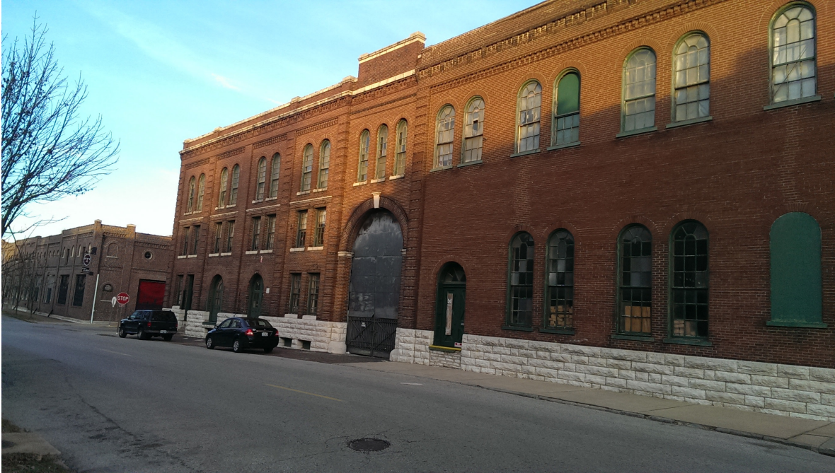
Figure 22: Rundown building on Lemp Ave. with destroyed and boarded windows (2014)
