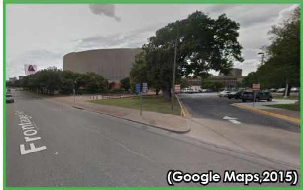
Figure 5-51: I-35 N Frontage Rd
