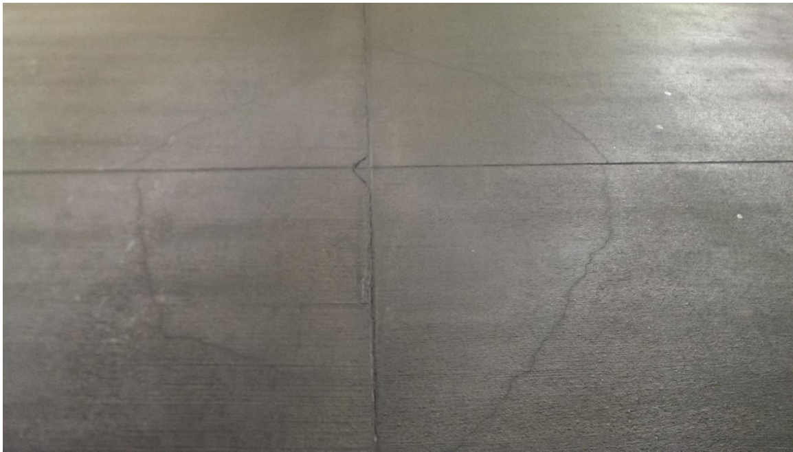
Figure 2-1 Pavement with Surface Cracks
