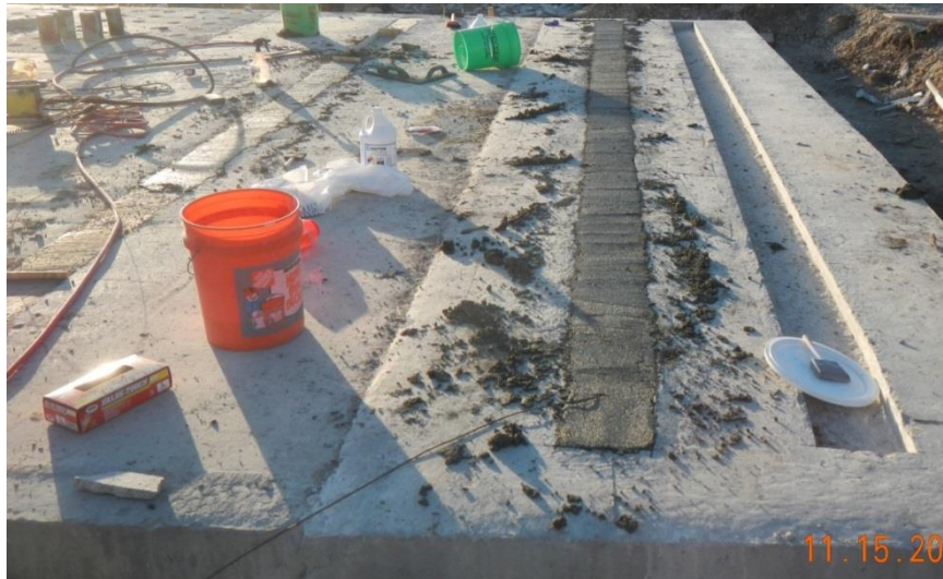
Figure 4.16 Repair Material Placed
