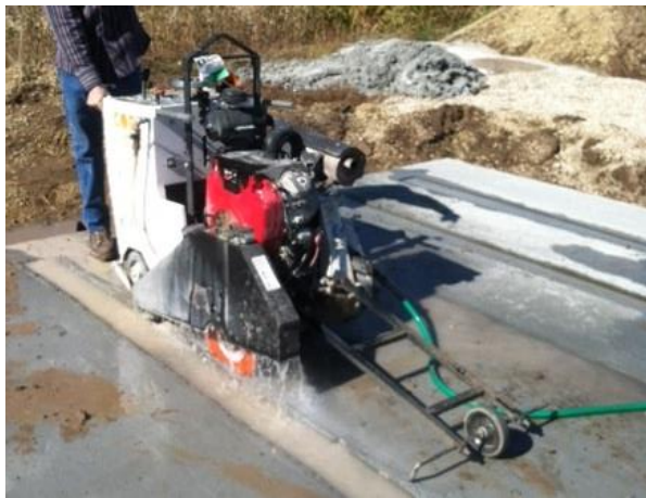
Figure 4.11 Saw Cutting Edges
