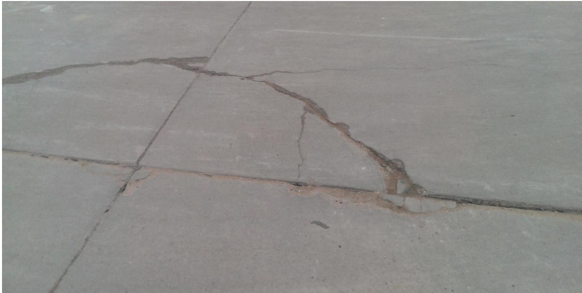
Figure 2-1 Pavement with Surface Cracks
