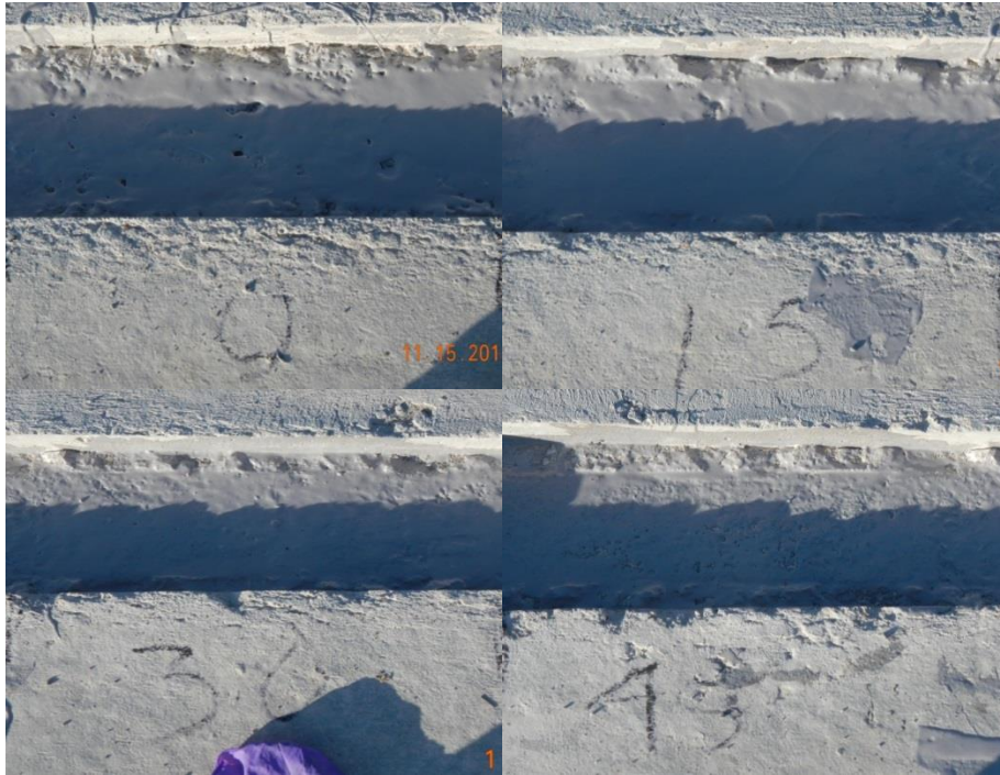
Figure 4.13 0,15,30, and 45 Minutes after Epoxy Bonding Agent Application
