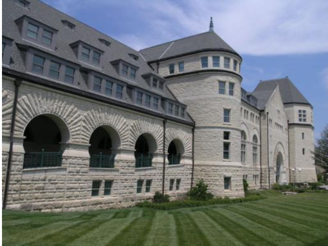
Figure 4.4 1997 renovation, south façade in Postmodern “Romanesque-Revival style” (Source: http://ksulib.typepad.com/talking/2007/12/k-state-keepsak.html . Last Accessed: 12-10-2013).
