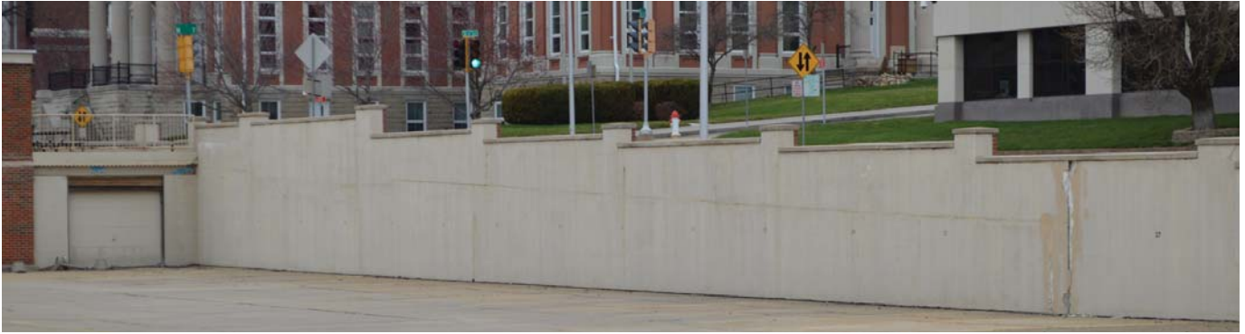
Figure 3.6: Existing Wall Looking Northwest (Prudenti 2014)
