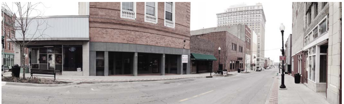
Figure 4.4: Stagnant Core (Albracht 2014)
