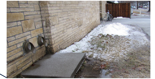
Topography change along the Northside of the building; winter rains and snowmelt refreezes creating sidewalk slipping hazards and erosion.
