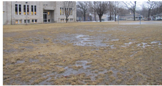
Location of temporary parking, compacted soil and flat topography causes water to pool.
