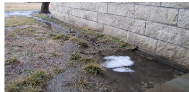
Erosion and pooling at the building foundation.
