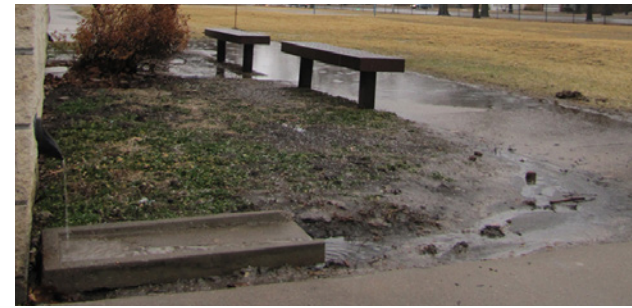
Erosion and pooling created by inadequate materials on ground plane and lack of slope away from school.
