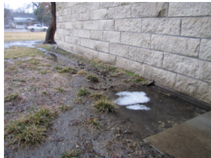
Potential foundation damage caused by erosion and pooling.
