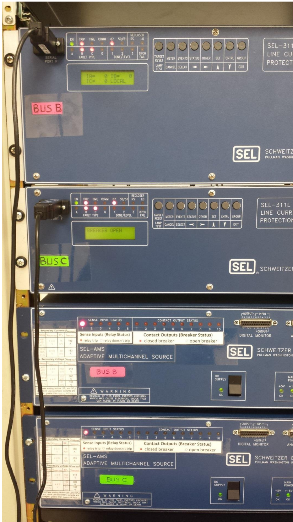
Figure 5.1 Front panel of relays and AMS for faults at A, B, and C
