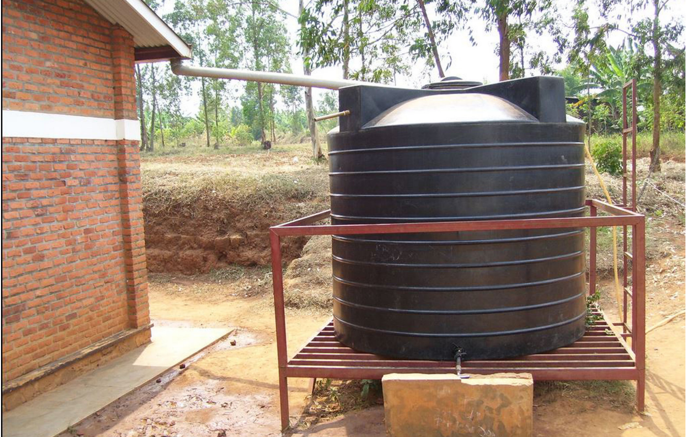
Figure 2.1 Modern Water Harvesting System Storage Container. (Image Source: Flickr user Bob Muller 2007)
