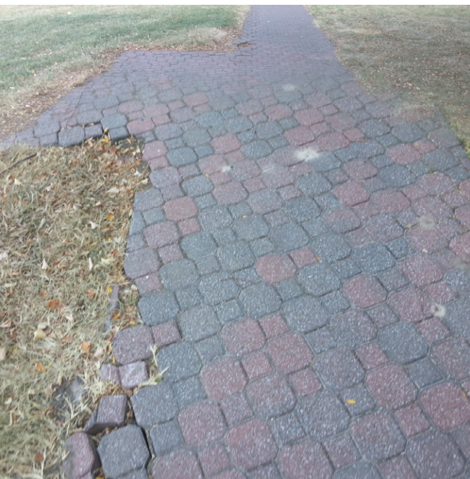
Figure 4.44 Paths are Poorly Maintained and Falling Apart
