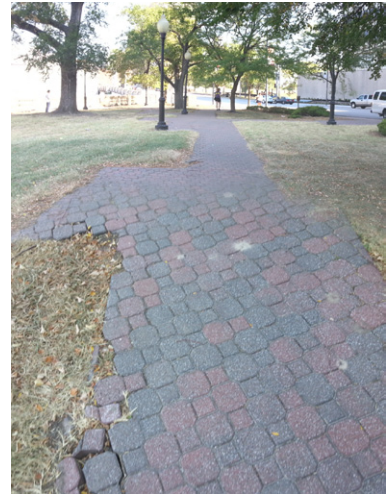
Paving in Poor Condition
