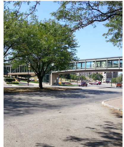
Skywalk over Pershing Drive
