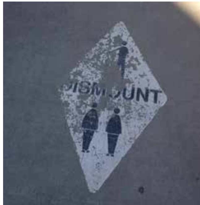
Figure 25 Current Condition of Pavement Marking, photo by John J. Scott (2014)
