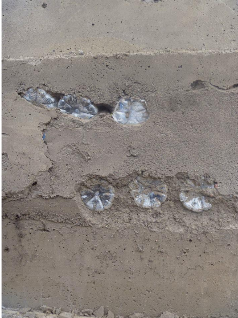
Figure 2.2 EWB Concrete Wall with Plastic Bottles, approval from Richard Kim
