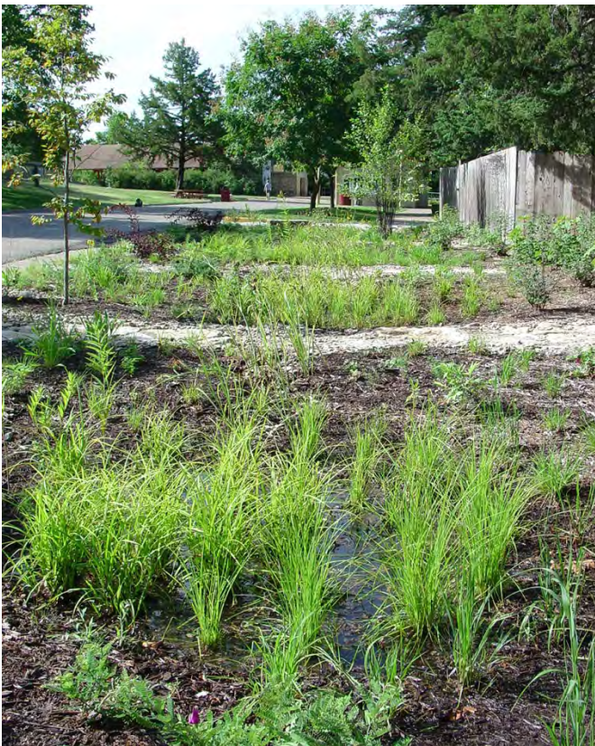
June 21, 2012 photos (lrs) of the pools less than 10 hours after a two-inch, four-hour storm event filled the pools. Infiltration works!
