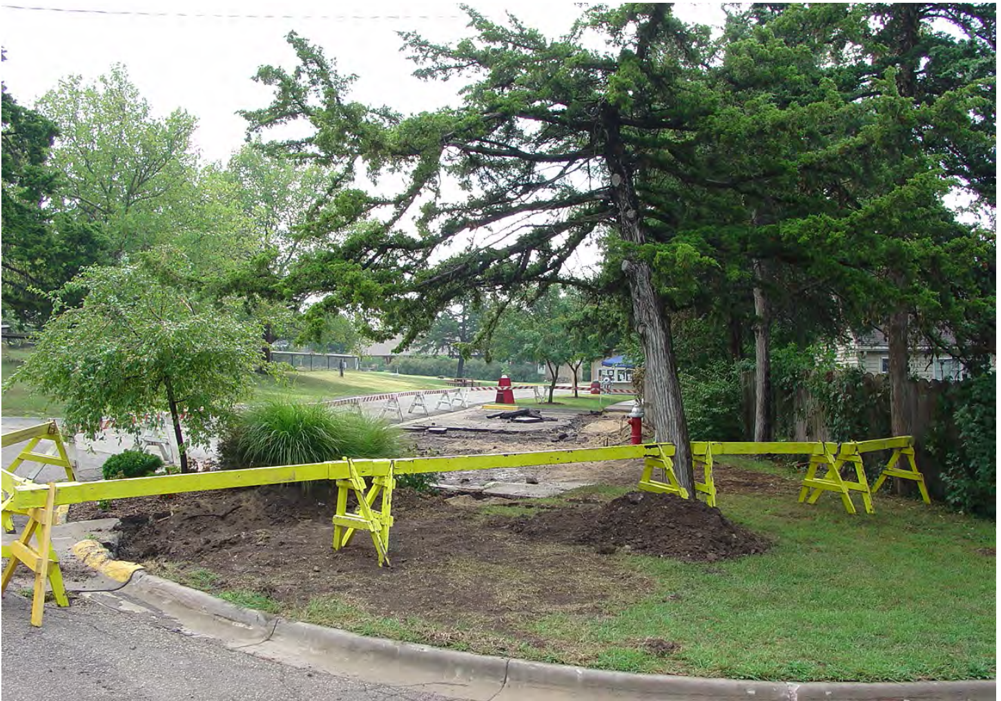
Photo by Lee Skabelund – August 30, 2011 during tear-out of impervious asphalt and concrete paving.
