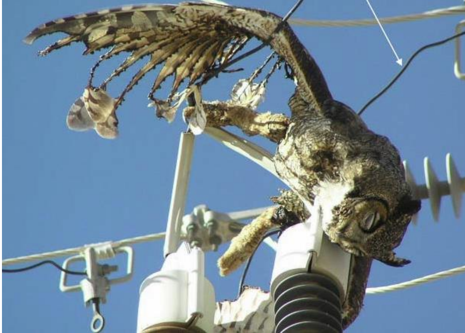
Figure 1.1 An Owl Caused Outage in the Distribution System [6] (With Permission of Rick Harness)
