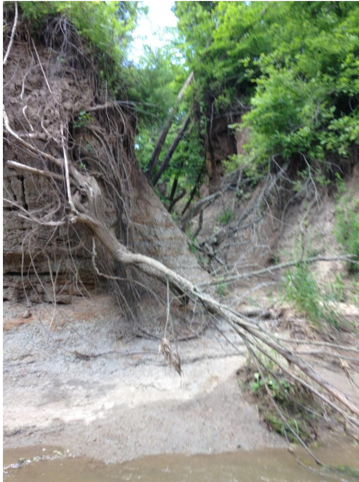
Figure 4.16 Image of gully side conveyance outlet
