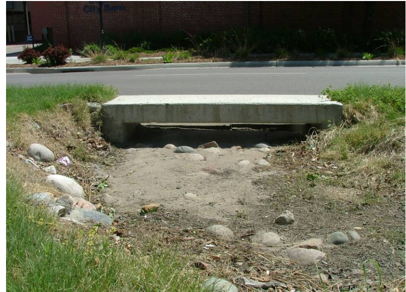
Figure 5-39: Sediment Buildup (Author)
