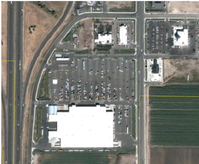
Figure 2-6: Aerial of typical Wal-Mart (Google Earth, 2006)
