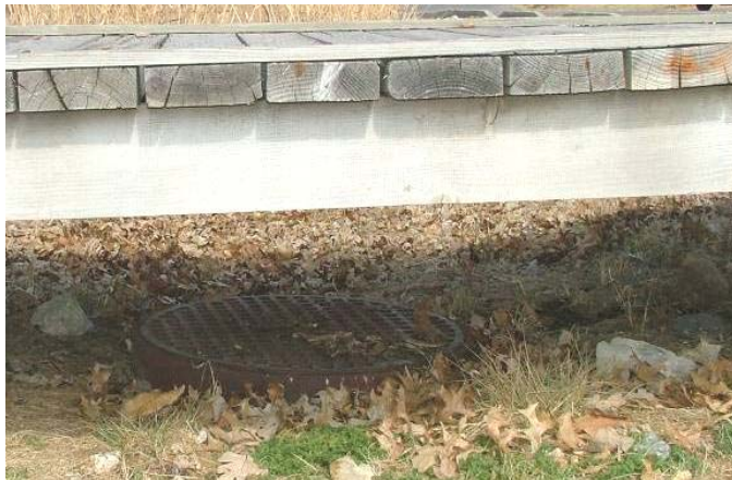
Figure 5-9: Overflow Inlet In The Middle of the Bioretention, at Hillcrest (Author)
