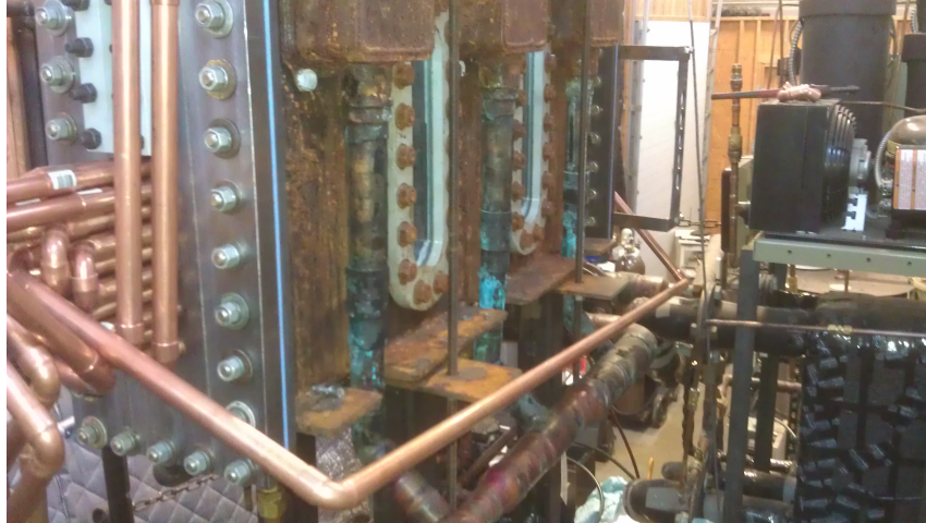
Figure 3.6: Picture of water channel A2 passing the outside of the test section. Picture is of dry-fitting stage with no insulation for clarity.
