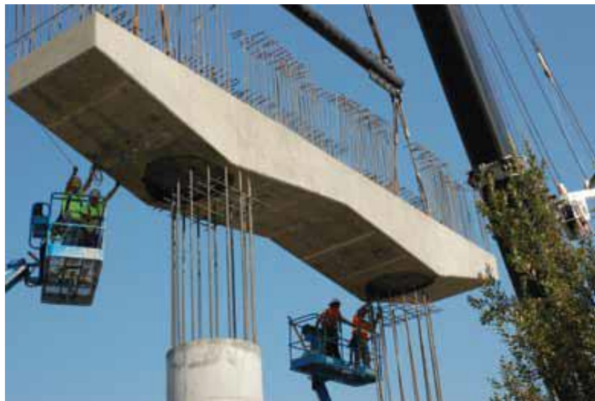
Figure 2.28: Placement of Precast Substructural Elements
