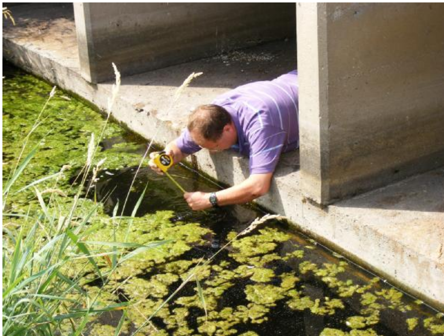
Figure 1.5: Scour Adjacent to Box Culvert
