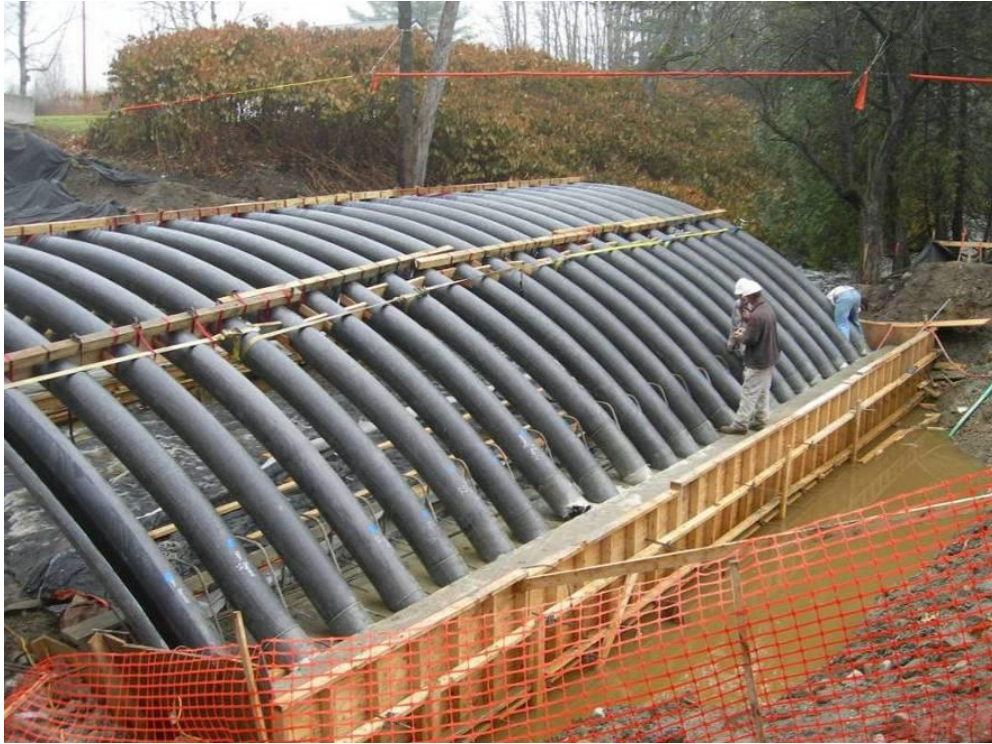
Figure 2.18: Bridge-in-a-Backpack Under Construction
