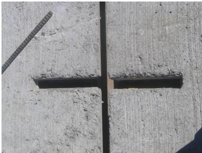
Figure 2.24: Rebar Connection for Adjacent Deck Panels*
