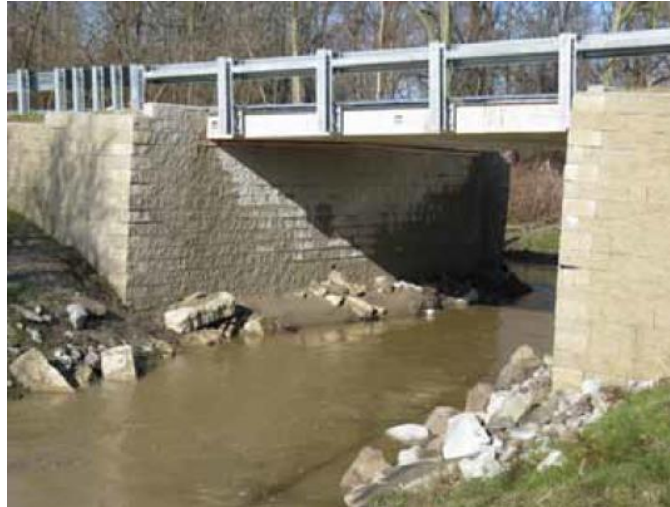
Figure 2.29: GRS Bridge System in Service
