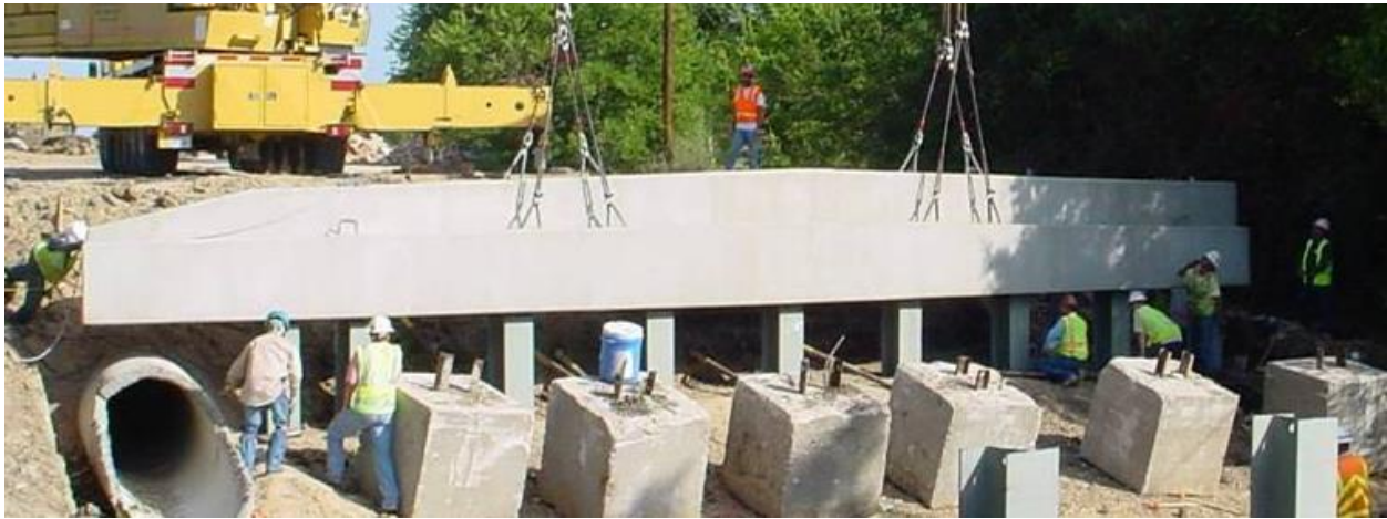
Figure 2.25: Precast Abutment Placed on Piles*
