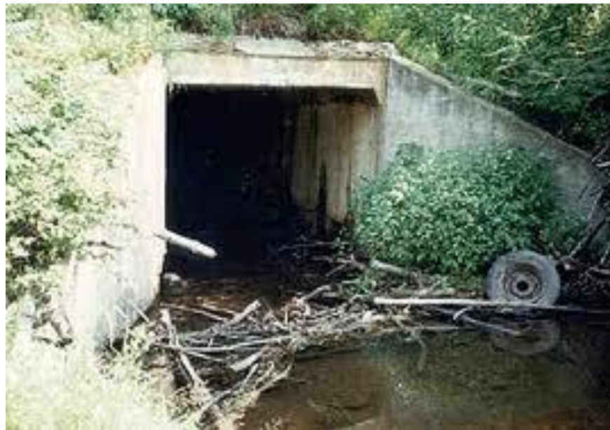
Figure 1.3: Box Culvert Obstructed with Driftwood
