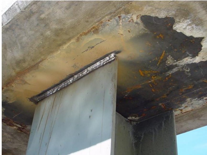
Figure 2.26: Welded Embedded-Plate Connection for Substructure*
