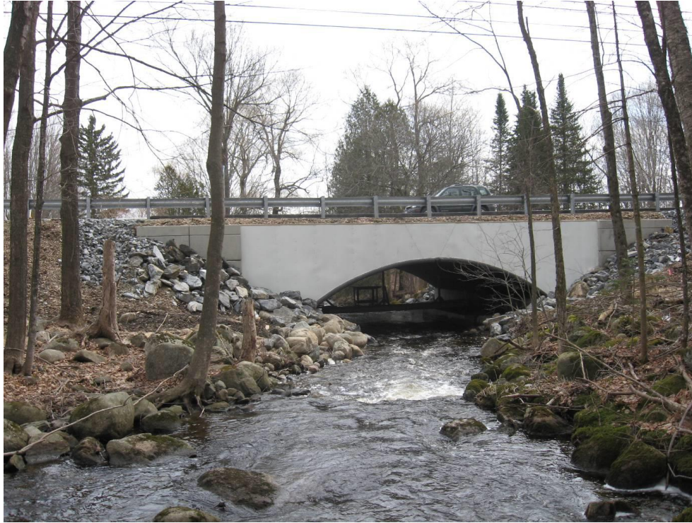
Figure 2.17: Bridge-in-a-Backpack
