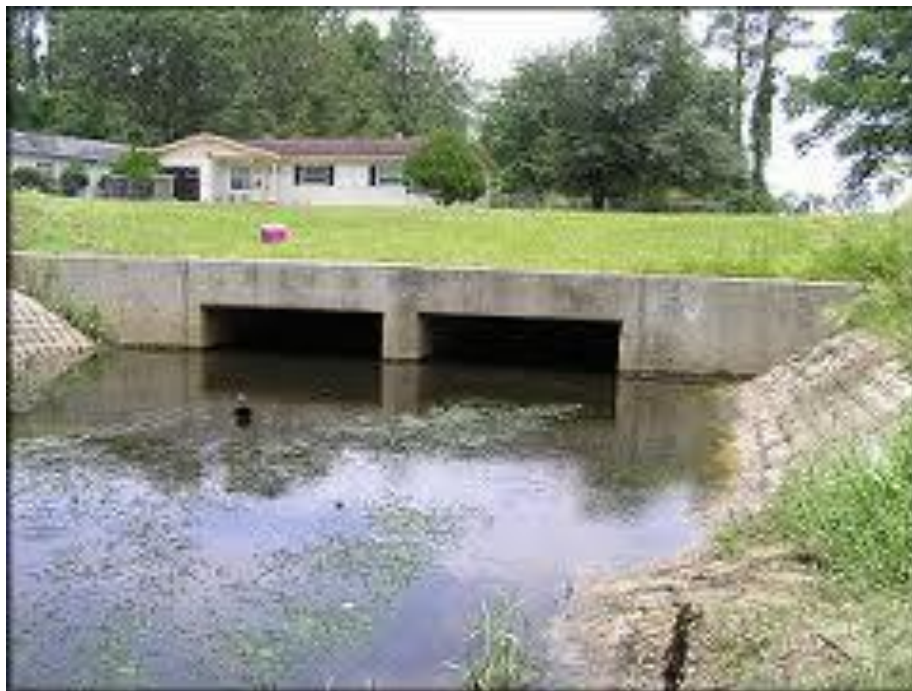
Figure 1.4: Box Culvert with Narrow Waterway Opening
