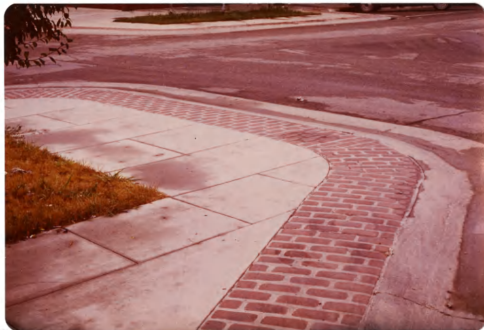
Figure 13. Sidewalks were outlined with a brick-patterned concrete edging.
