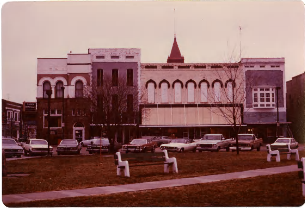
Figures 9 and 10. Typical examples of the results of the storefront renovation project in Red Oak.
