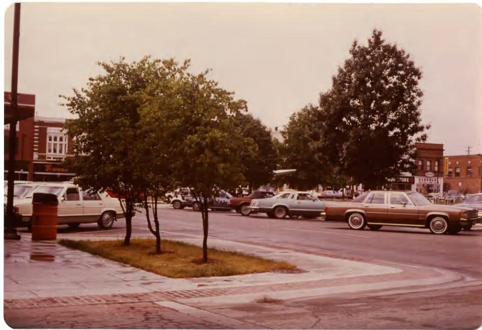
Figure 12. Curbs were extended at the corners and at mid-block points to allow for planting areas and to increase pedestrian safety.
