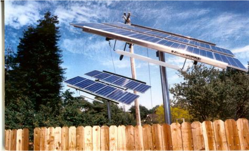
Figure 2.3: Pole mounting with tracking
