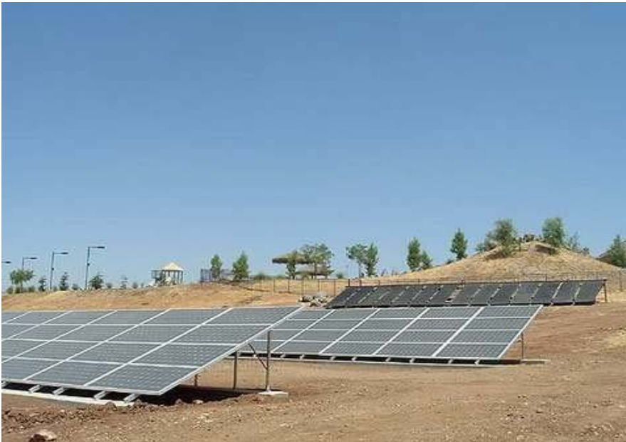
Figure 2.4: Ground mounting with metal leg base
