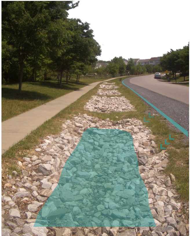
Figure 28: Infiltration Trench Diagram. Diagram by author. Adapted from Sustainable Stormwater Management, 2007.
