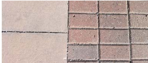
Figure 5.18 (Photo by author) Brick edging along sidewalks adjacent to 700 Merchant
