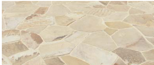
Figure 5.19 Irregular limestone pavers
