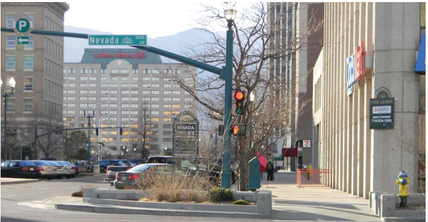
Figure 1-26. View of pedestrian bump out at Pikes Peak and Nevada Avenues (photo by Devin Ash)
