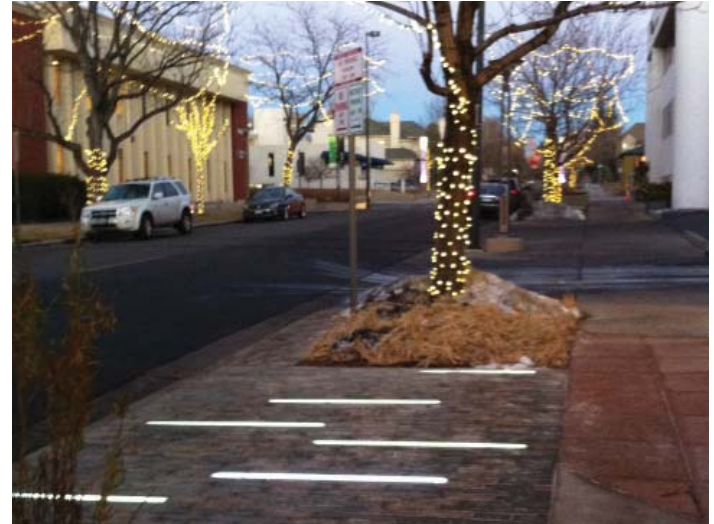
Figure 2-8. LED lighting strips in pedestrian zone (photo by author)
