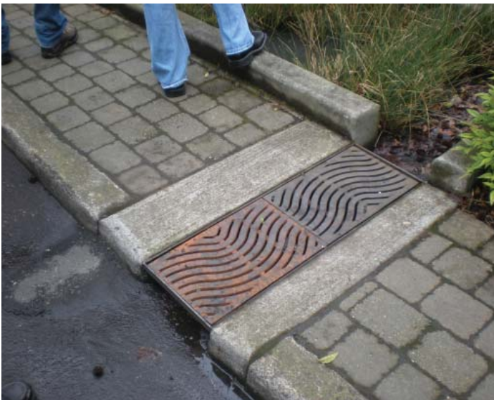
Figure 2-13. View of curb chase (photo by author)
