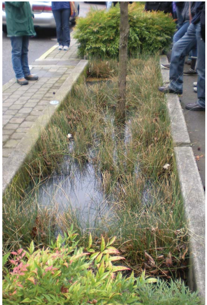
Figure 2-15. View of stormwater planter (photo by author)
