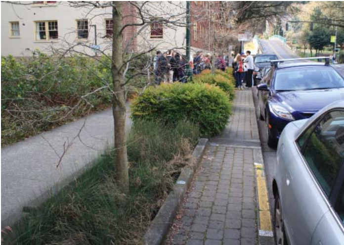
Figure 2-16. View of main sidewalk zone, stormwater planters, and parking egress zone (photo by Glen Jarrett)
