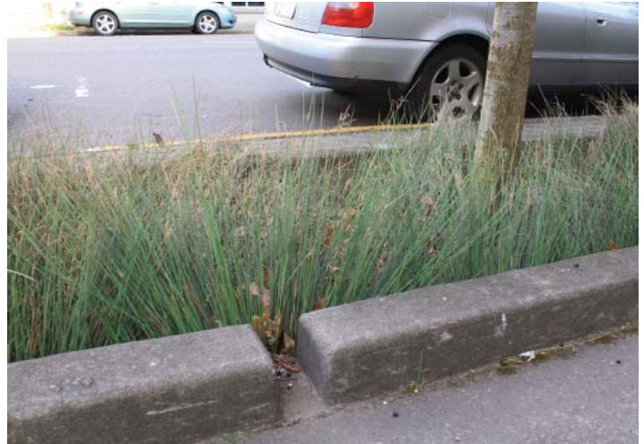
Figure 2-17. Narrow curb cut directs runoff from the sidewalk into the planter (photo by Glen Jarrett)
