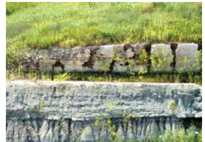
Figure 3.17—Summer Road cut in Manhattan, KS
