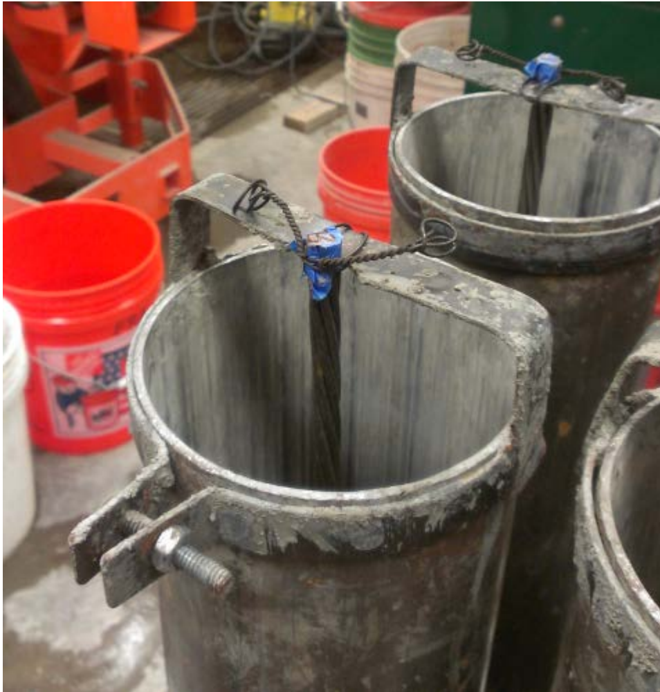
Figure 5.3 Additional fixture used to center strands during casting
