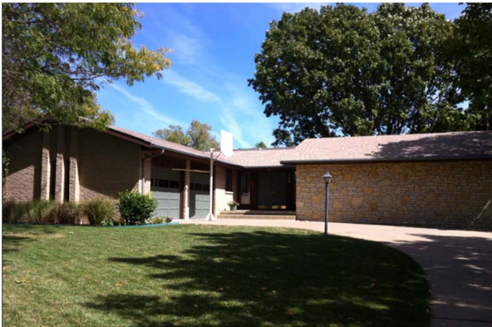
Figure 1-1 Photograph of the Residence Being Analyzed
